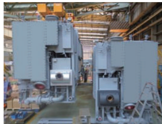
Setting both chillers onto common base
